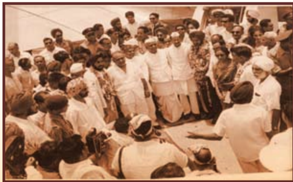
Historic Reception at Palam Airport
